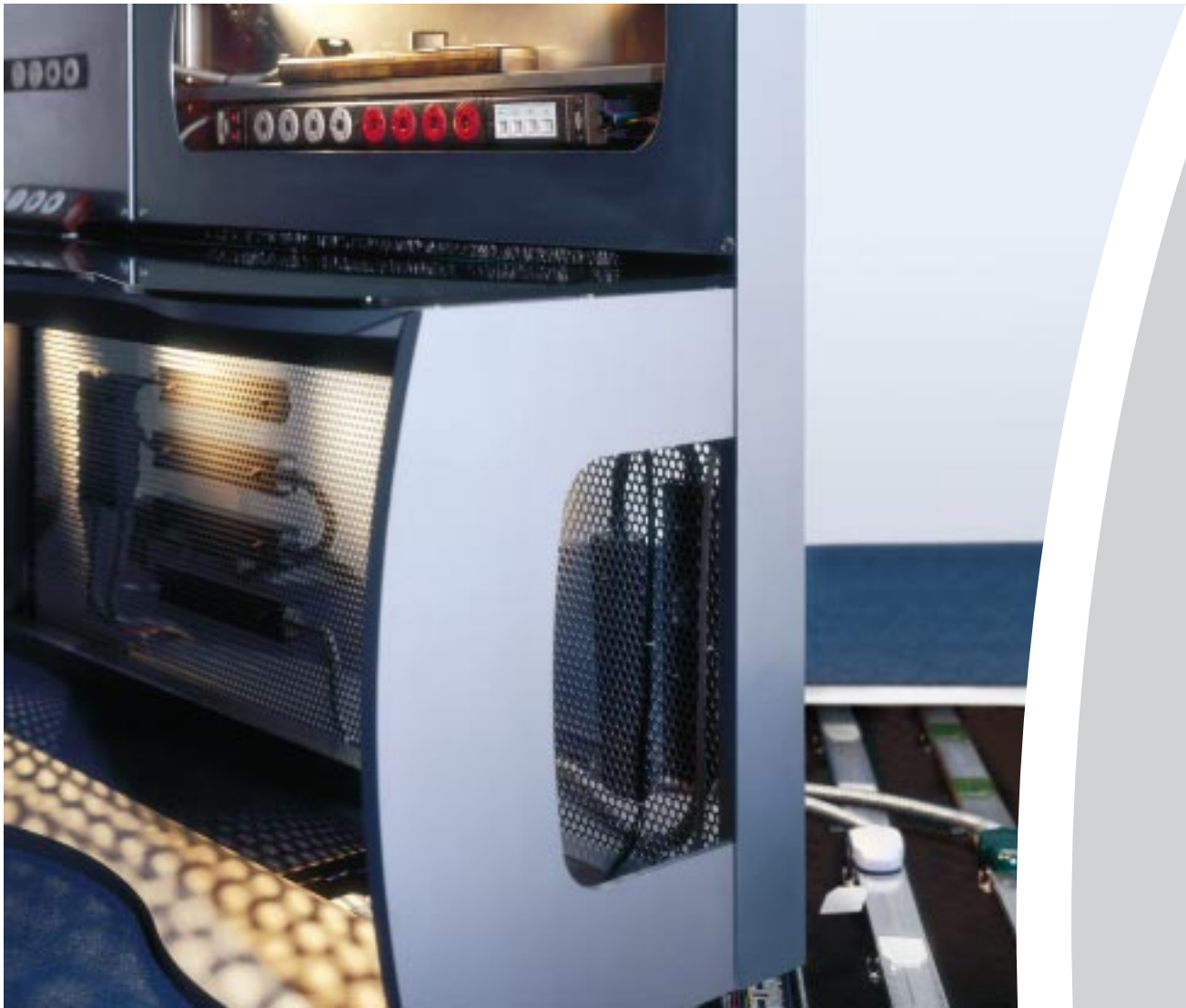
Rotasoc power units connected to underfloor power track system
