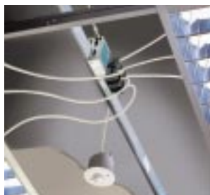
Lightrak Busbar Trunking and EIB Lighting Control System
